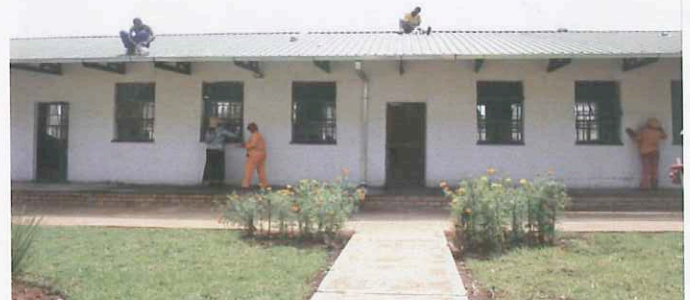
The school after it was renovated and painted
