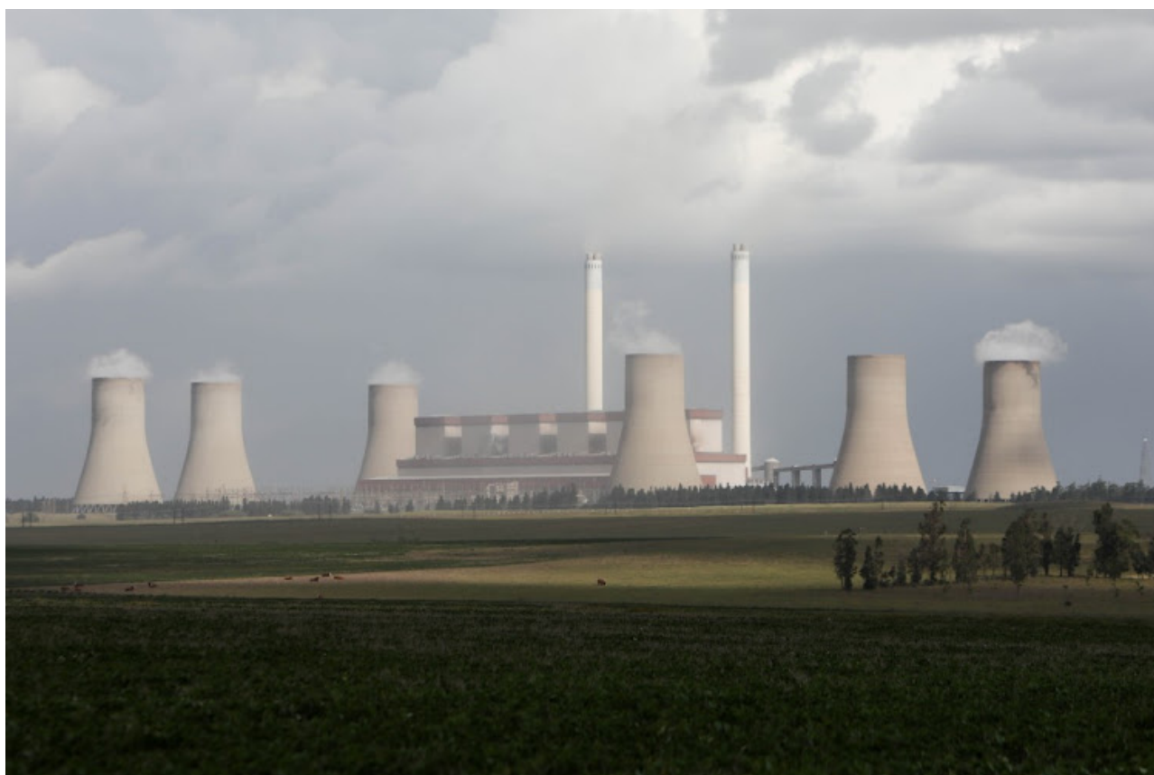
Tutuka Power Station in Standerton, Mpumalanga, January 25 2023. Picture: SUPPLIED
