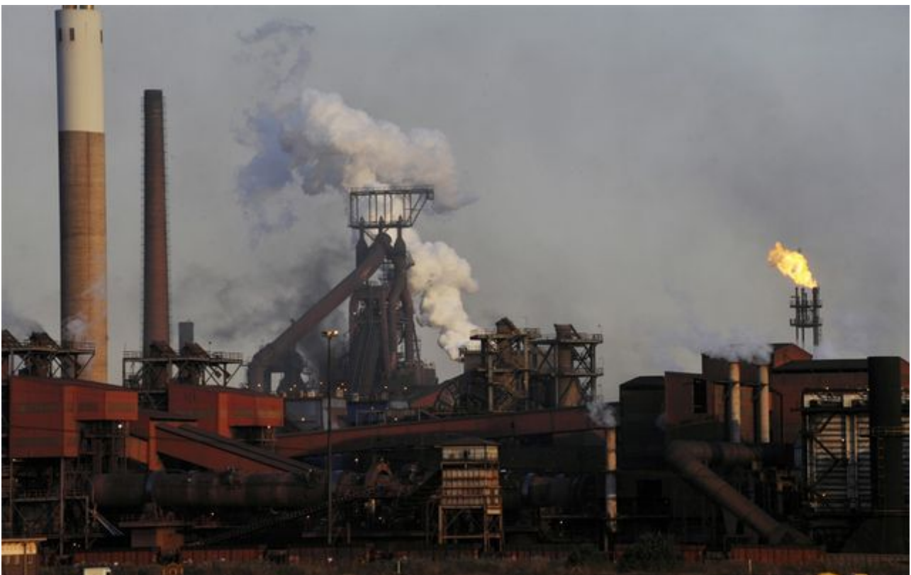
ArcelorMittal SA's Vanderbijlpark plant. Picture: FINANCIAL MAIL
